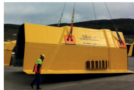
GRP cover design and test lift.
